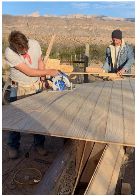
Our crew replacing the siding on the clinic building in January.
