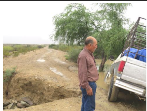
Pastor Pepe gets stuck trying to go around the hole created by heavy rains the night before.
